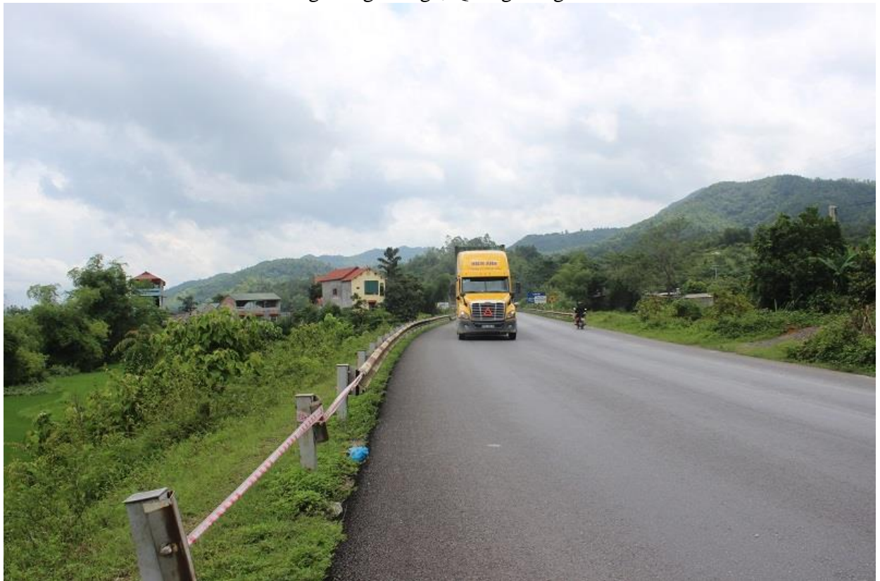
National road 1A running through Khun Phang village, Quang Lang commune
